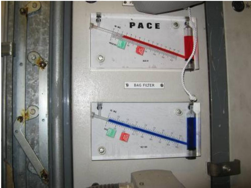
**Figure 3 Most manometers on site are well calibrated**
