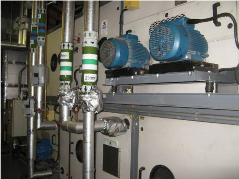
**Figure 1 AHU insulation to pipework in good condition**
