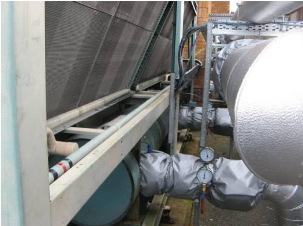
**Figure 2 Chiller pipework well insulated**
